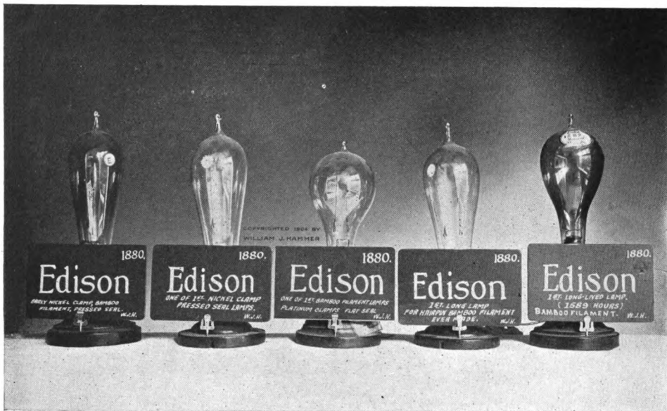
Fig. 10 Standard "Pear shaped" Edison lamps of 1880
