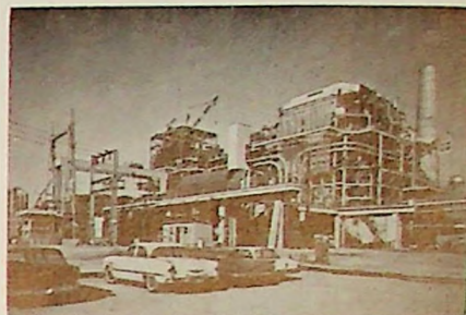
ETIWANDA STEAM STATION UNITS 3 & 4
