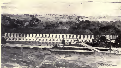
Power House The Canadian Niagara Power Company
