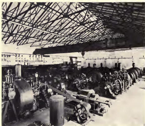
Interior of Station No. 2 The Niagara Falls Power and Manufacturing Company
