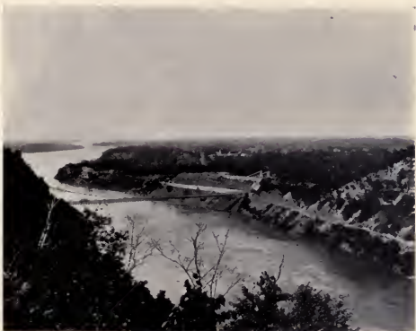
The Suspension Bridge Across Niagara River at Lewiston
