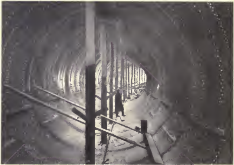
Interior of Pipe The Ontario Power Company
