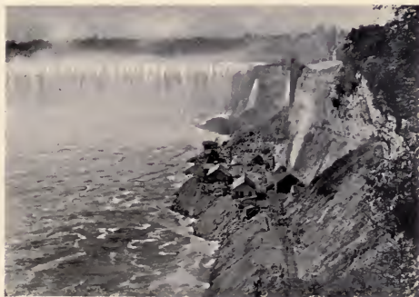
Site of Power House The Ontario Power Company
