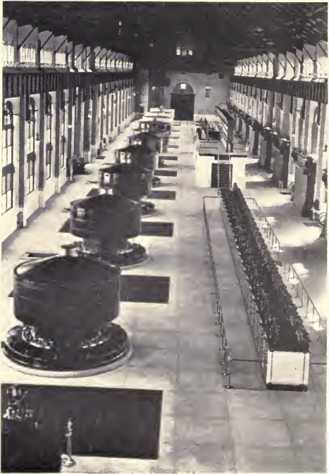
Interior of Power House No. 2 The Niagara Falls Power Company
