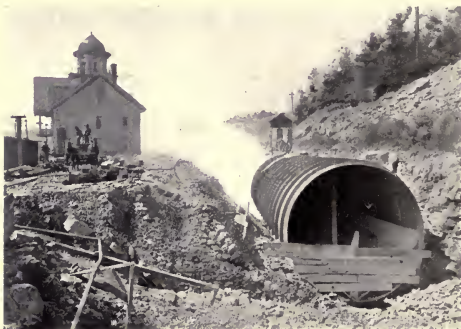
Sand Blasting the Pipe The Ontario Power Company
