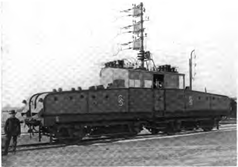
FIG. 25.— EXPERIMENTAL SIEMENS' HIGH-VOLTAGE LOCOMOTIVE.
