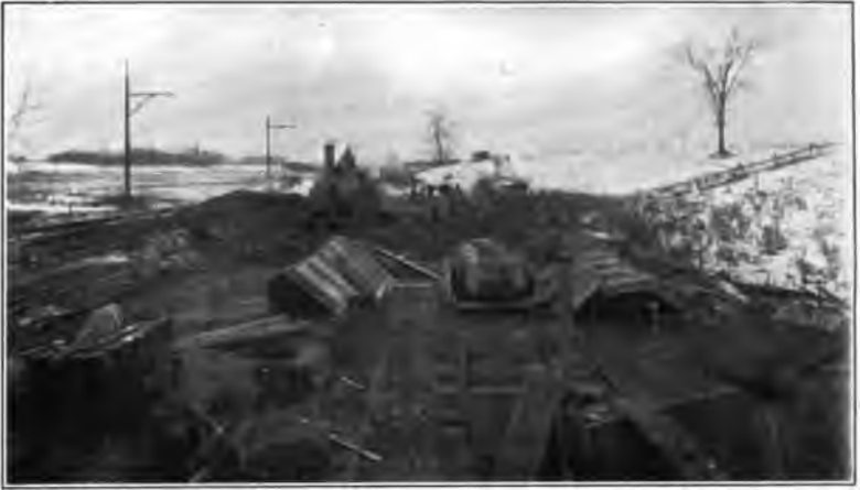
FIG. 12.— VIEW OF CARHOUSE SITE AFTER FIRE WHICH DESTROYED LOCOMOTIVE NO. 1.
