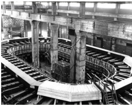
Alpha Racetrack of Y-12 Electromagnetic Plant where uranium isotopes were separated to enrich uranium used for the bomb
