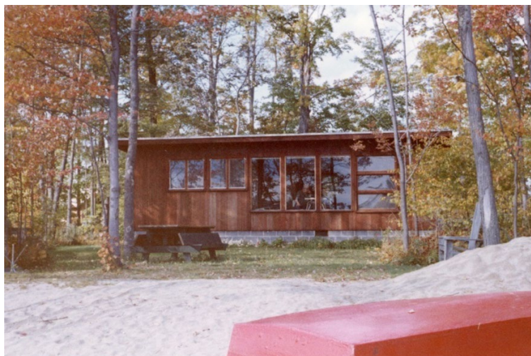
Cottage (back of photo indicates it was developed in Oct 1962)
