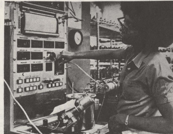
FINAL EFI FUEL FLOW TEST
