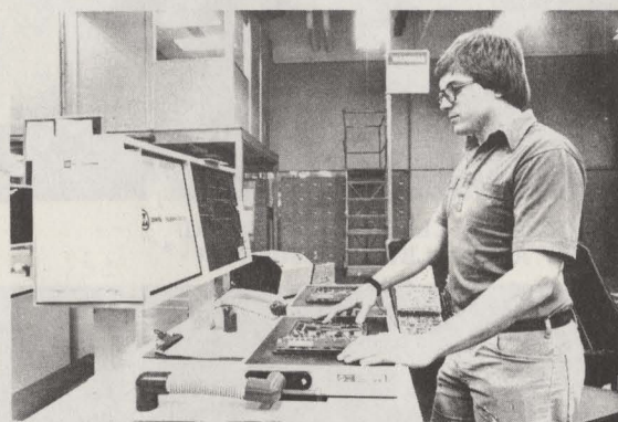
"BED OF NAILS" COMPONENT PARTS PRESENCE TESTER
