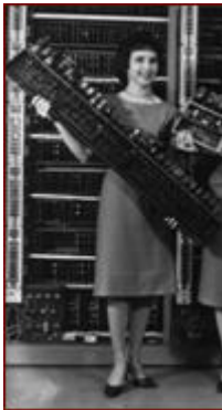
Figure 2. The ENIAC decade ring counters (Source: US Army Photo)
