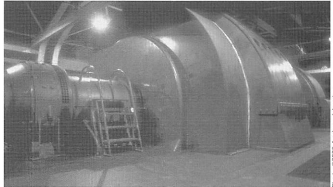
Figure 9. One of the rotating frequency converters at Richmond Station.
