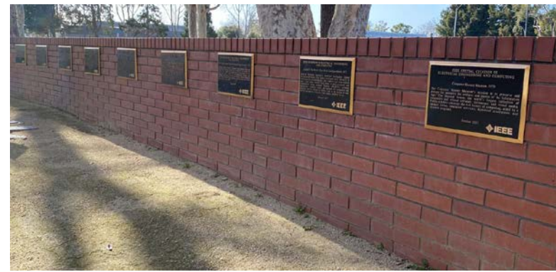
Duplicate: CHM Front Brick Wall (in place now)
