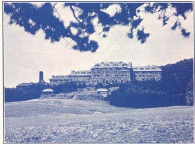
Grove Park Inn Convention Headquarters
