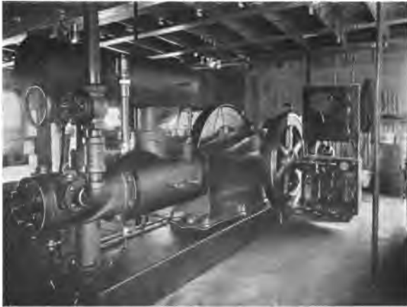
Interior of Compressed Air Station
