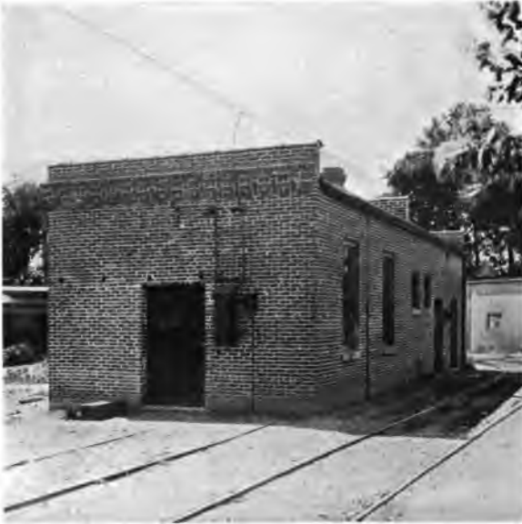
Compressed Air Station
