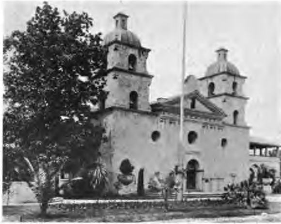
California State Building
