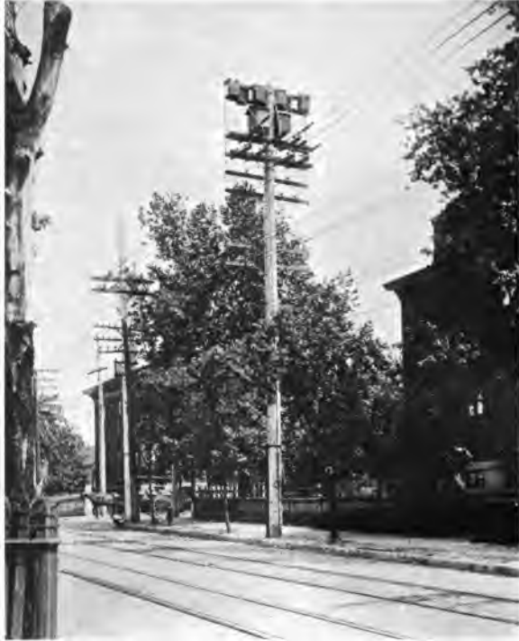
Terminal Poles—Garrison and Franklin Avenues
