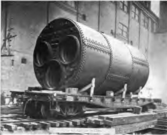
Marine Boiler—Ashley Street Plant
