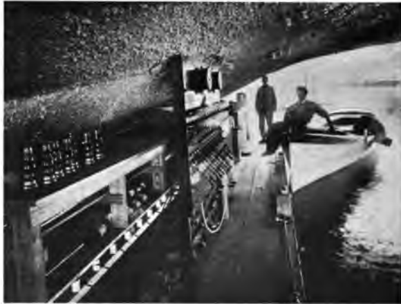
Charging Station, Electric Launches
