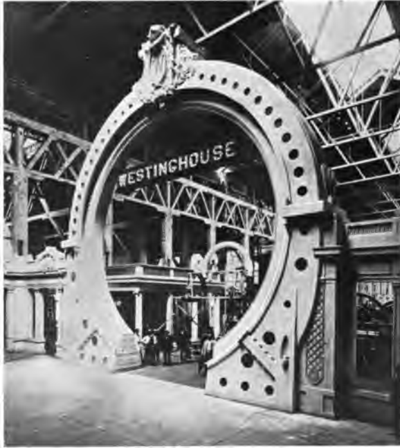
Entrance to Service Plant
