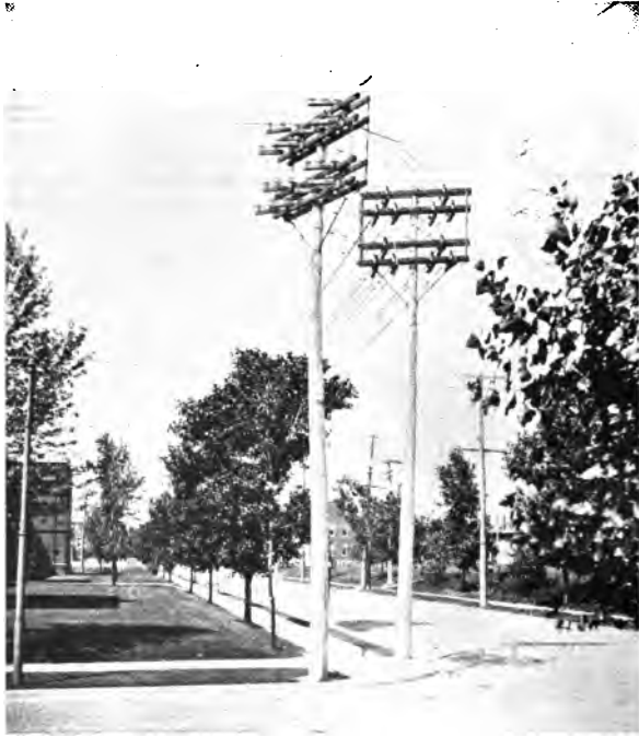
Corner Construction—Lake and McPherson Avenues
