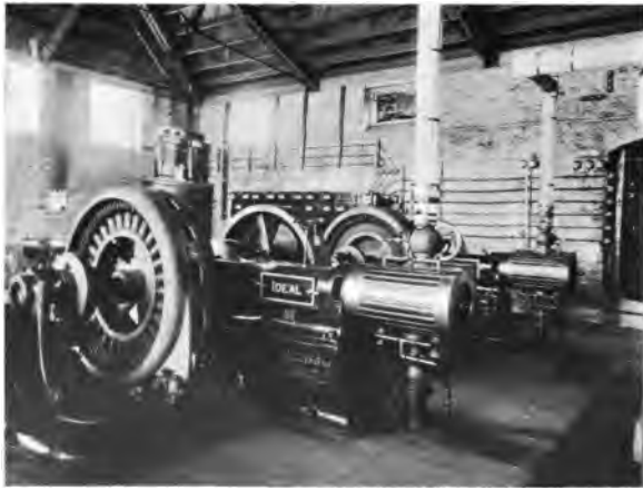
Interior of Power House
