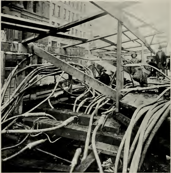
After fire, cables brought to surface and spliced
