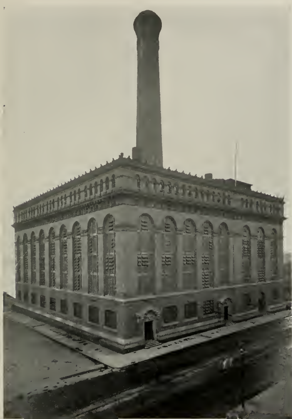
Ninety-Sixth Street Power Station
