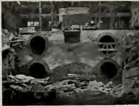
A section of the condensing tunnel construction
