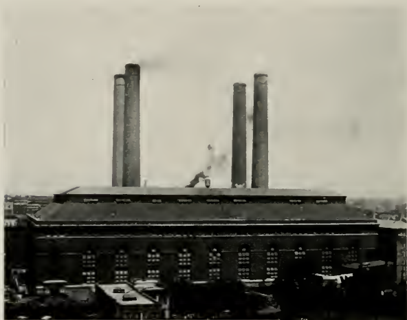
74th Street Power Station, Manhattan Division
