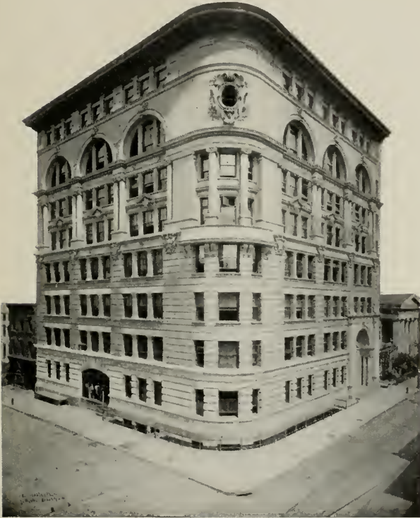
General Offices of New York and New Jersey Telephone Company, No. 81 Willoughby Street, Brooklyn, N. Y.
