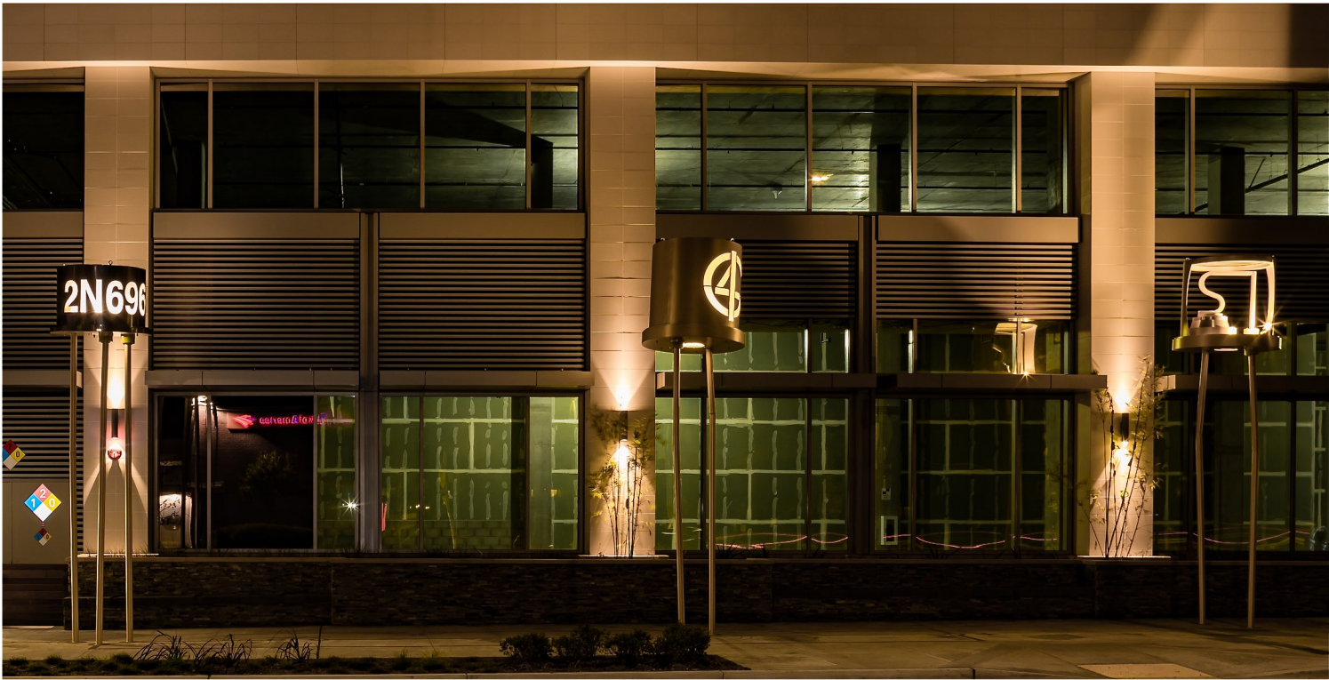
Night View. Installed Silicon Diode and Transistor Sculptures and etched sidewalk Circuit Board, 391 San Antonio Road, Mountain View, CA
