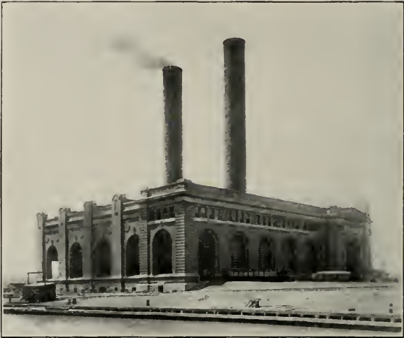
FISK STREET POWER HOUSE COMMONWEALTH ELECTRIC COMPANY
