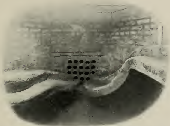
REPRESENTATIVE CONDUITS AND MANHOLE, SHOWING ISOLATION OF CABLES
