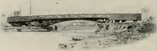
ASHLAND AVENUE BRIDGE, CLOSED
