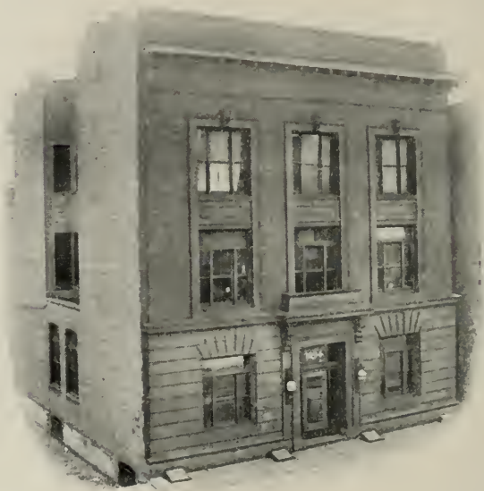
WEST MADISON STREET SUBSTATION
