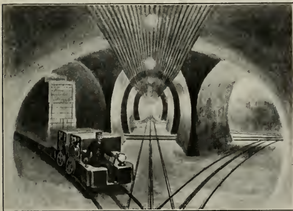
STREET INTERSECTION OF TUNNEL
