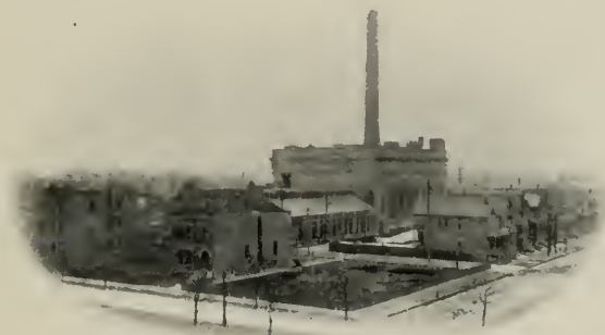
EXTERIOR OF THE FIFTY-SIXTH STREET STATION
