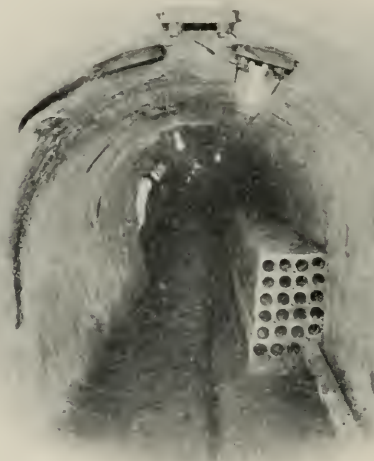
TUNNEL CONSTRUCTION AND CABLE PROTECTION
