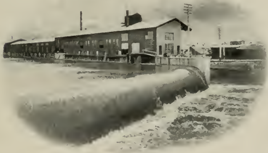
POWER HOUSE AND DAM, ECONOMY LIGHT AND POWER COMPANY
