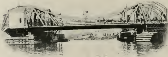
CLYBOURN PLACE BRIDGE, CLOSED
