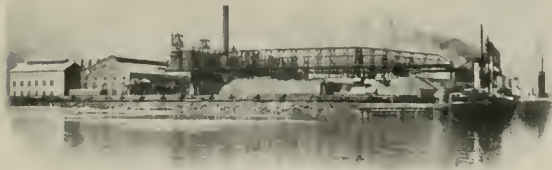
ORE BRIDGE, SOUTH CHICAGO
