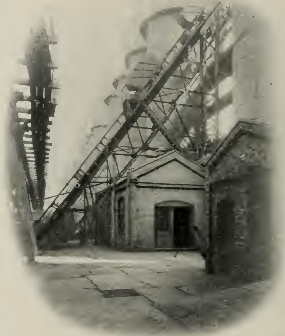
SKIP HOIST, ILLINOIS STEEL COMPANY
