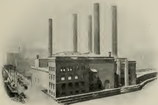
EXTERIOR OF HARRISON STREET STATION
