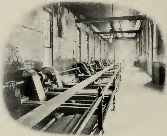
INTERIOR OF BRIDGEPORT PUMPING PLANT
