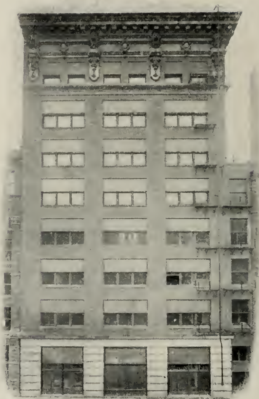
MARKET STREET SUBSTATION BUILDING
