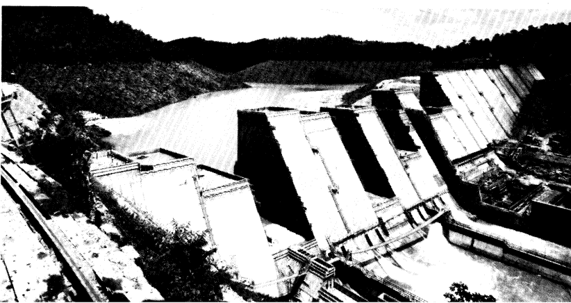
Norris Dam, started in 1933 and completed in 1936, was the 1st dam built by TVA TVA
