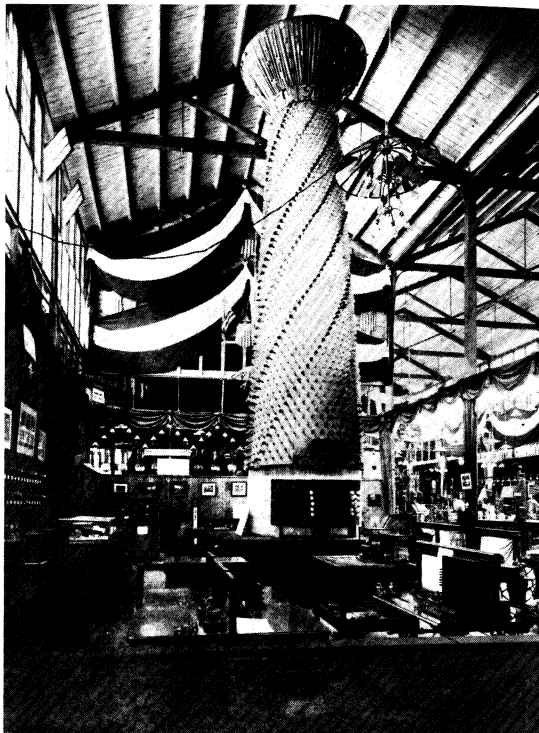
Edison National Historic Site
