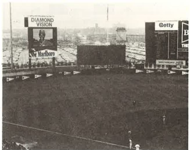
Fig. 10 7.3 x 10.9 m screen, installed April 1982, New York Mets Shea baseball stadium
