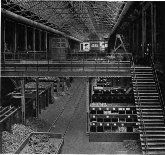
Central Aisle of Machine Shop
