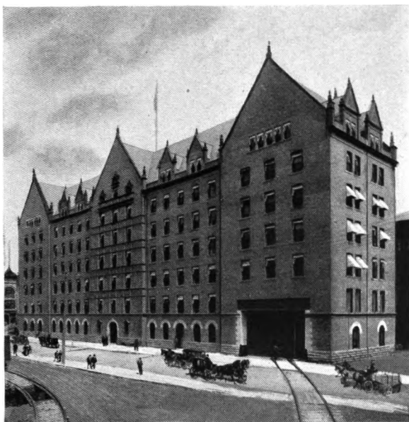
Main Office Building, Westinghouse Electric & Mfg. Co.
