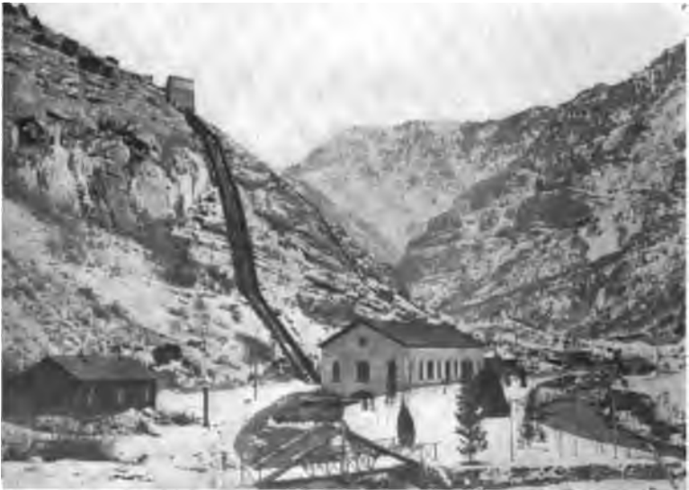
FIG. 6.— THE LOGAN POWER-HOUSE.
