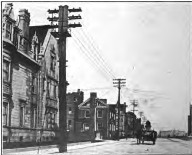
FIG. 12. CABLE POLE CONNECTING OVERHEAD AND UNDERGROUND LINES. II — 679
