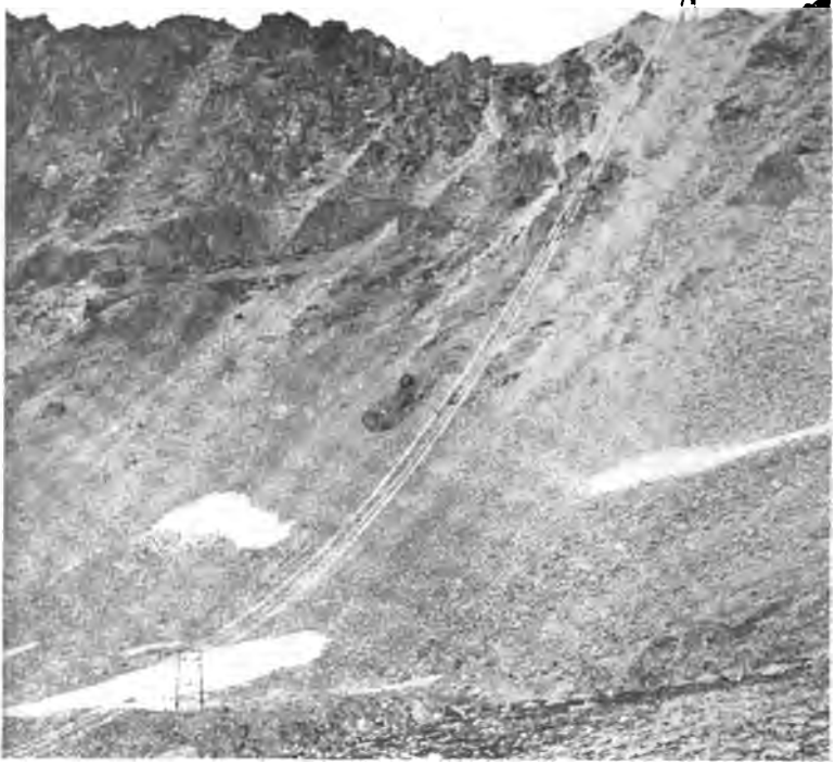
FIG. 4.— LONG SPAN AT CAMP BIRD DIVIDE.
