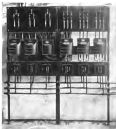
FIG. 4. TWO- AND THREE-WIRE METER INSTALLATION.
