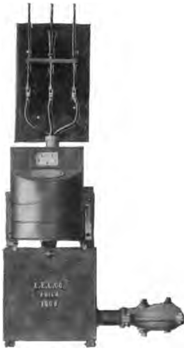
FIG. 2. SINGLE METER INSTALLATION.
