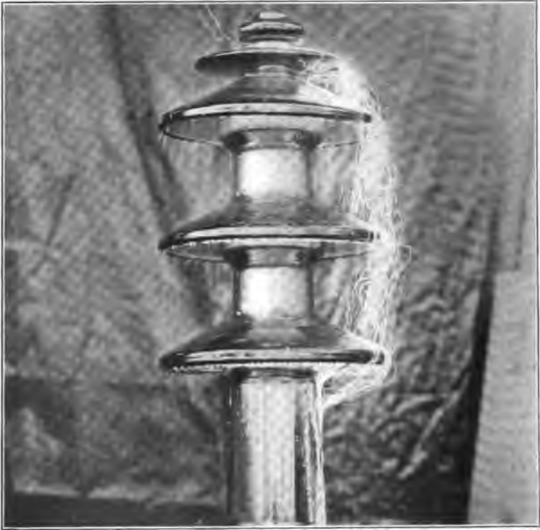
FIG. 13. EXPERIMENTAL INSULATOR UNDER TEST AT 198 KILOVOLTS.
