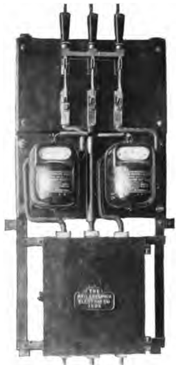
FIG. 3. INDUCTION METER INSTALLATION.
