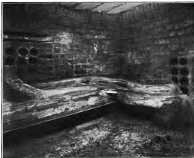
FIG. 9. PROTECTING CABLES IN MANHOLES WITH SPLIT-CLAY TILE.
