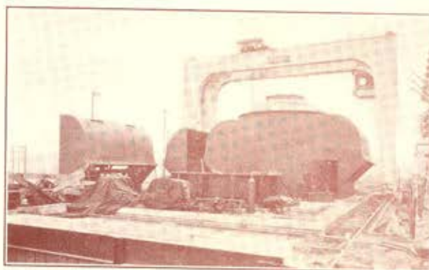
Leaside Station—25,000 kv-a. Outdoor Condensers
