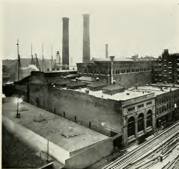
Exterior, Atlantic Avenue Station
