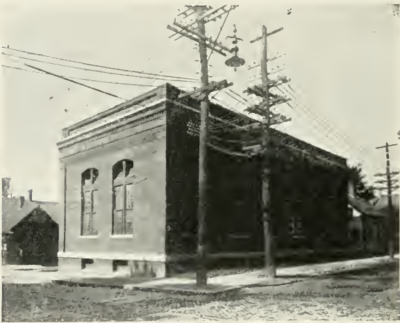
Exterior, Brockton Sub-station
