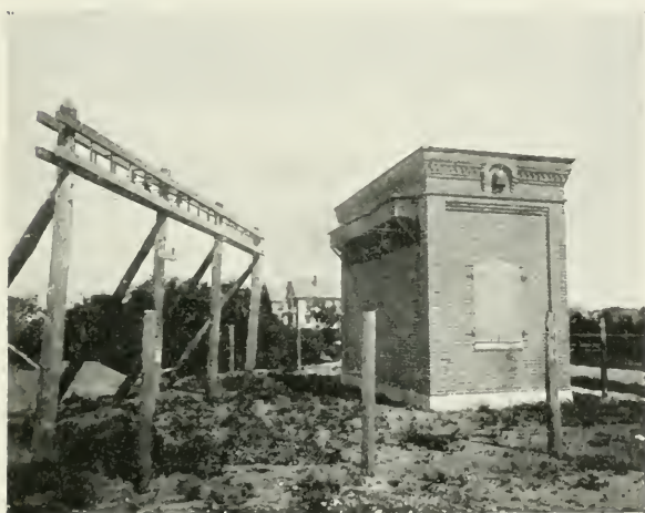
Cable Terminal Station, Brockton
