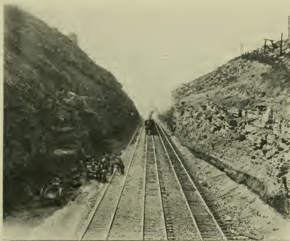
Enlarging a Deep Cut for a Fourth Track
