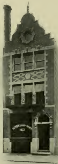
One of the Substations
