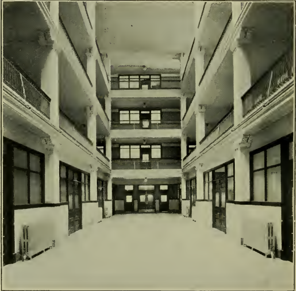
Corridor at Main Exchange
