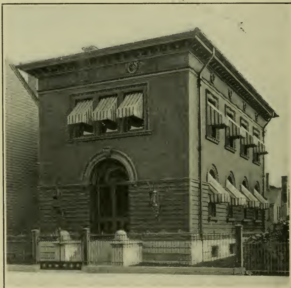
IV. Gas Testing Station, Philadelphia
