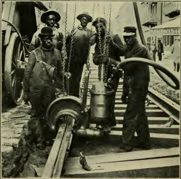
Electric Riveter Fastening Rails together
