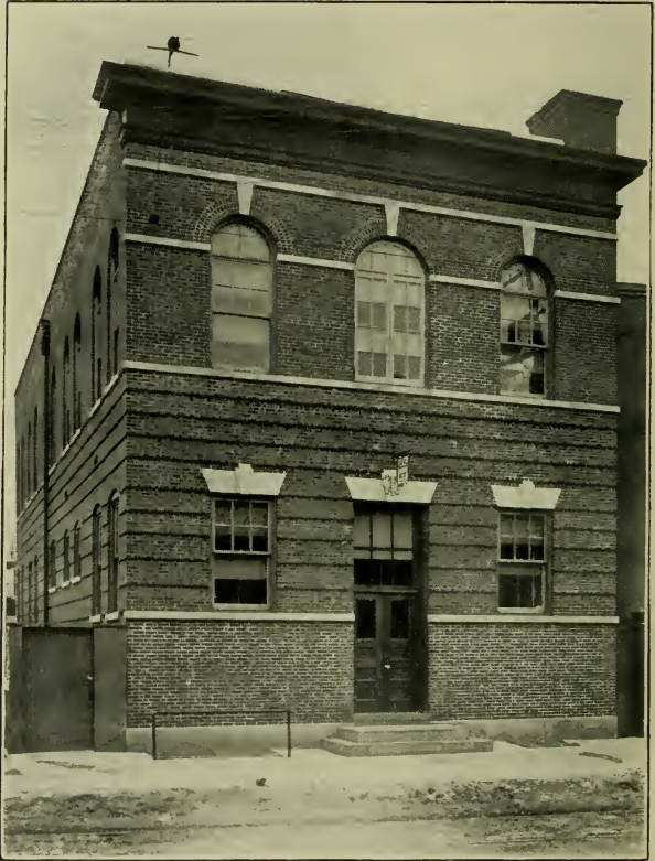
East Exchange, Kensington Avenue, below Somerset Street
