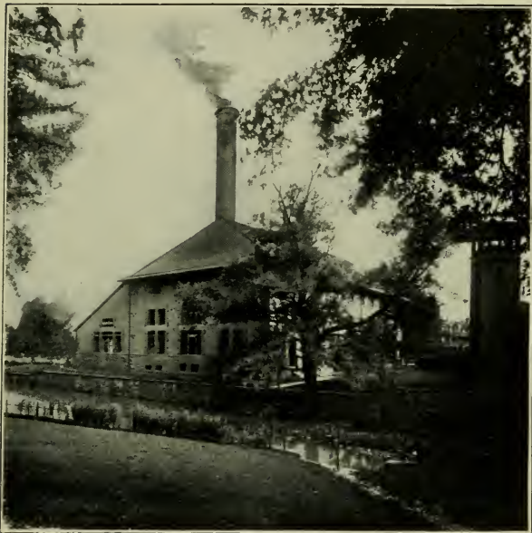
Power House at Ogontz which Furnishes Power for Operating the Cars to and from Willow Grove, on Old York Road
