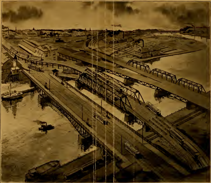
Showing the New Steel Bridge over the Schuylkill River which will carry the Train-Cars as they Emerge from the Subway, over an Incline to the Elevated Tracks which Extend from Thirtieth Street-Schuylkill River-to the County Line, a Distance of nearly Four Miles. To the Left is the Present Market Street Bridge, which will Carry the Present Surface Road Cars
