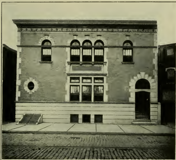
Sub-office Station of the Philadelphia Rapid Transit Company on Germantown Avenue near Erie Avenue
