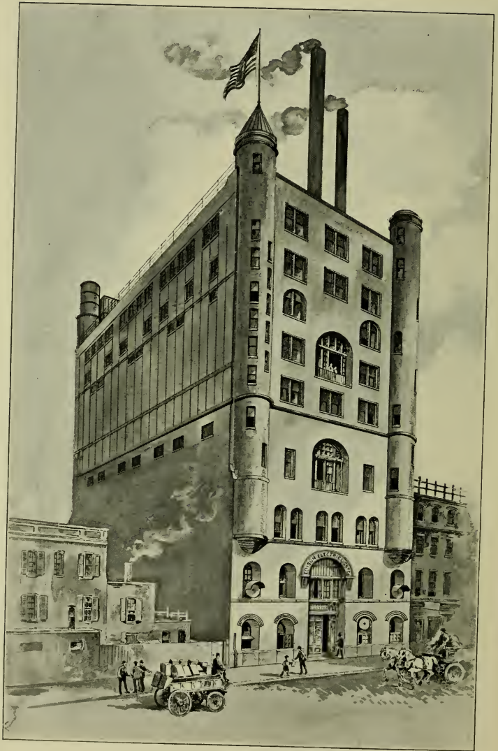
Direct Current Generating Station
