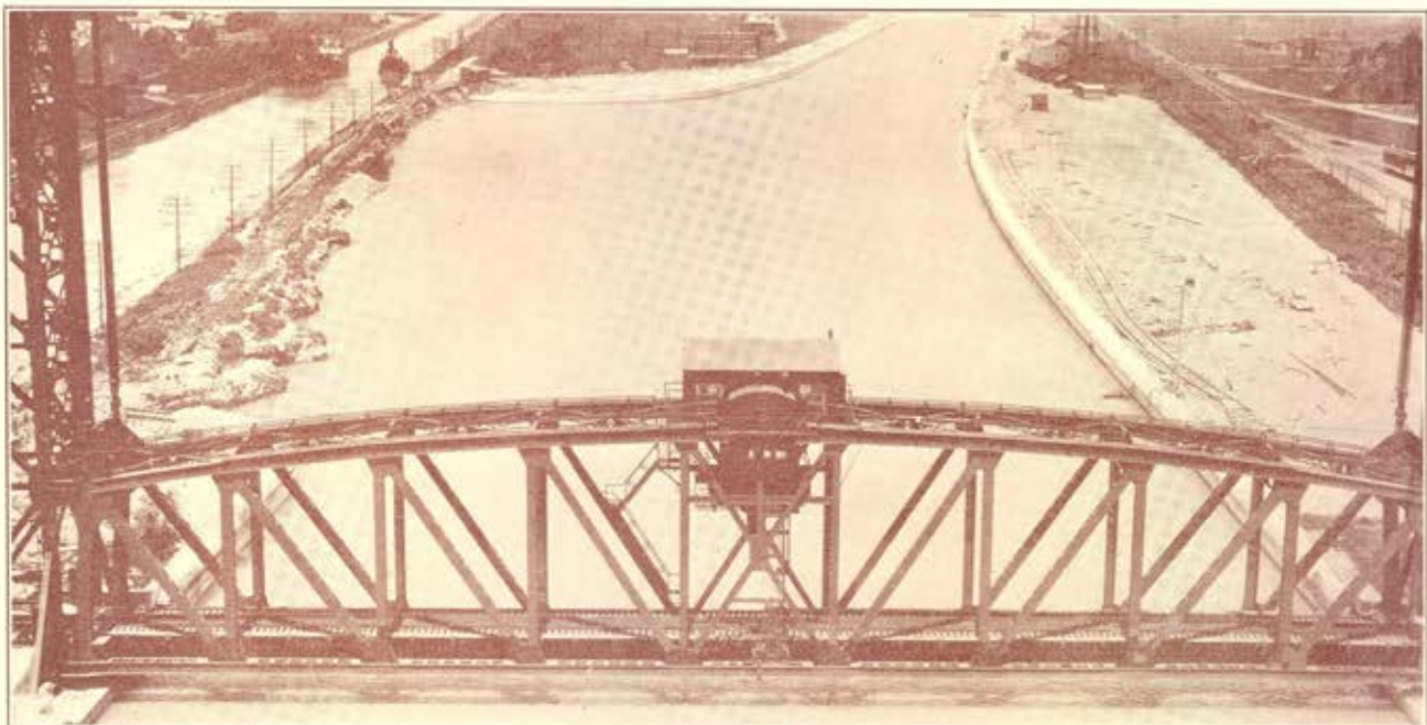
Welland Canal at Lift Bridge
