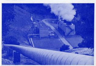
Geysers Power Plant—America's first geothermal power plant, a property of Pacific Gas and Electric Co. This unique plant utilizes natural steam from the bowels of the earth to generate electric power.
