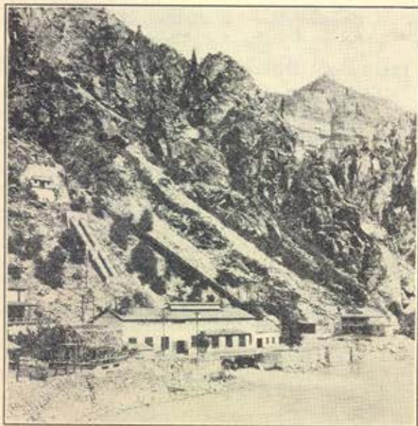
SHOSHONE POWER PLANT
