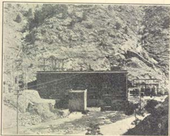
BOULDER CANYON HYDRO PLANT
