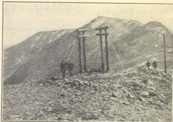
DENVER-SALT LAKE TELEPHONE LINE CROSSING THE CONTINENTAL DIVIDE
