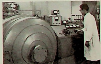
Wesgo vacuum processing furnace for oxide free brazing alloys
