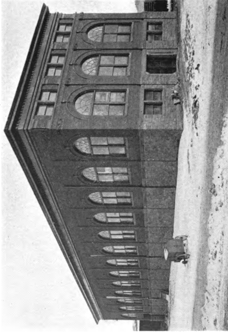
Dock Street Sub-Station, Schenectady Railway Company
