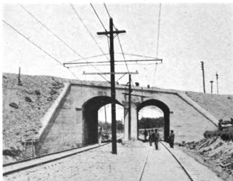
Concrete Bridge—Ballston Division
