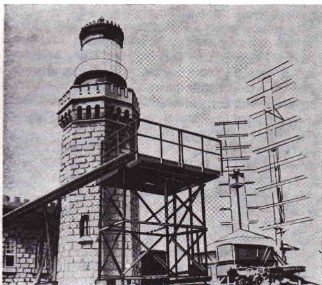
Early models of both the SCR-270 and SCR-271 installed at Twin Lights, New Jersey, about 1940.
