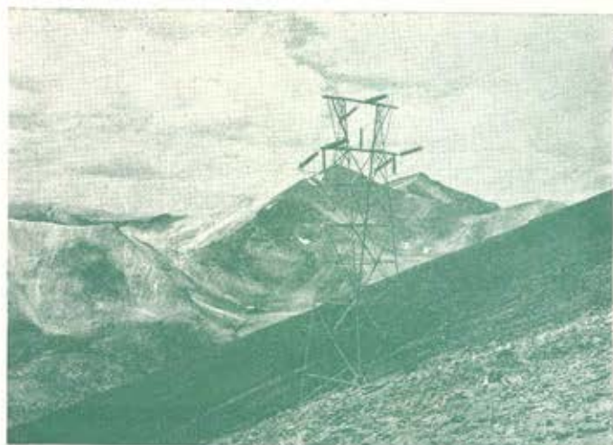
100-Kv Line of the Public Service Company of Colorado Near Argentine Pass (altitude 13,500 ft.), Where the Lightning Investigation at Higher Altitudes Was Conducted
