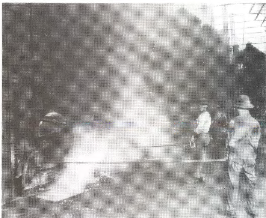
Figure 1. Gas manufacturing plant in Denver for the first street light in 1880. Removing coke after the coal was "baked" to produce combustible gas.
