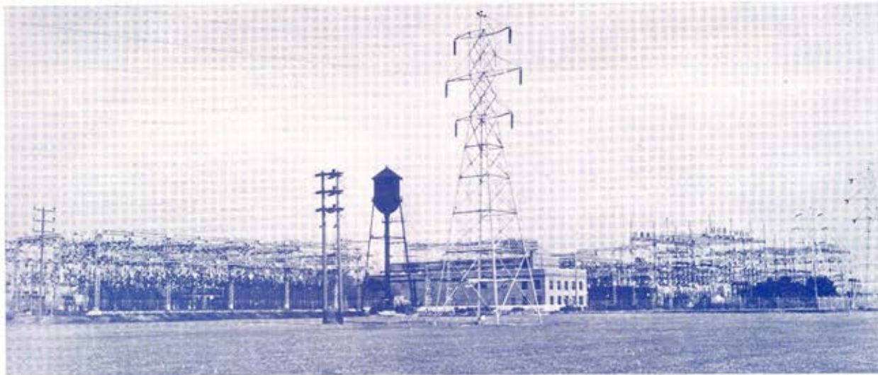
Lenore Substation of the Public Service Company of Indiana
