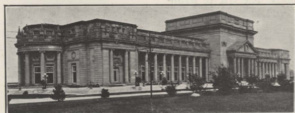
Power House of Toronto Power Company Containing Eleven 100,000 Kv-a. Generators
