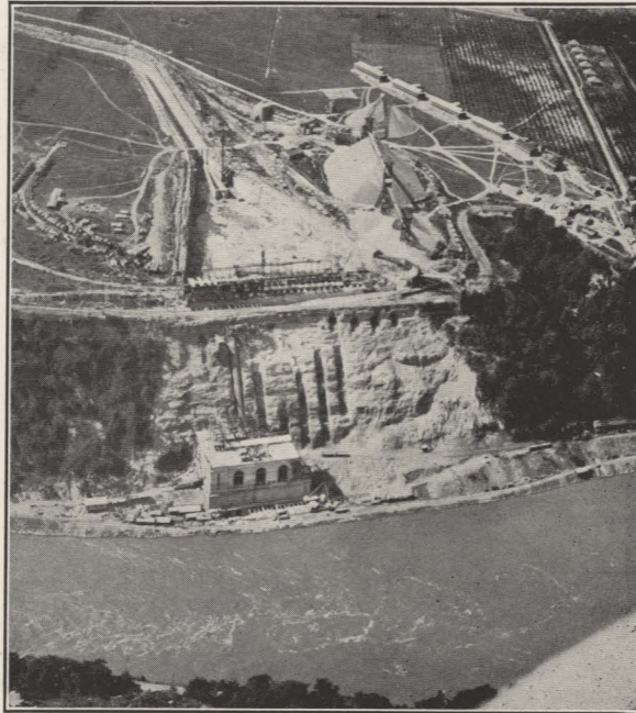
Queenston Power House, Penstocks, Head Gates, Forebay and Canal in Construction
