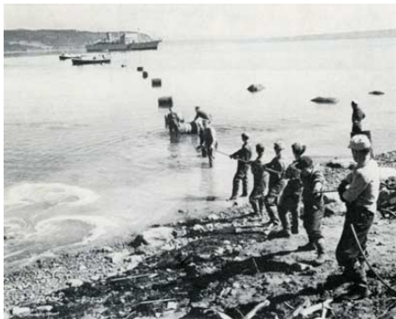
At Clarenville, Newfoundland, cable end is floated on drums and pulled ashore from the ship.
