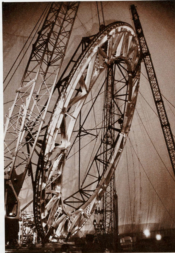
Cranes lift a 70-foot wheel (below) into vertical position. The wheel weighs in at 40 tons and will be used to point a huge antenna for experiments in satellite communications, which will begin with the launching of a Telstar experimental satellite this spring. The construction project is for Bell Labs., and protected from the winter by an inflated shelter seen overhead.
