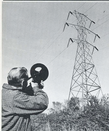
'Corona hunter' — Aiming an ultrasonic "gun" at a high-voltage transmission line, W. E. Pakala, Westinghouse power engineer, tests the line for electrical leakage. If present, the corona produces ultrasonic sound waves which are received by the device and made audible through electronic circuitry.
