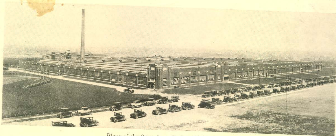
Plant of the Stromberg-Carlson Tel. Mfg. Co.
